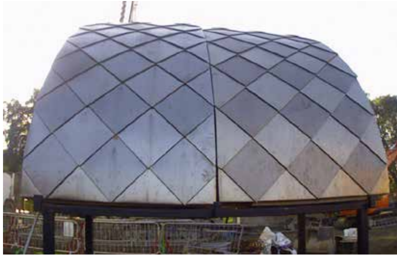
Image 01 Two Mock Ups North Facing on Site
